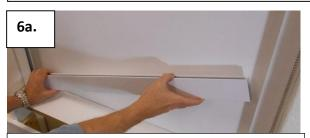
For easier installation, slide light blocking brush up and out of the way while installing the bottom channel.
